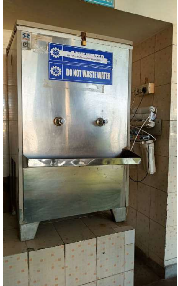
Potable Water, Water Cooler With Ro System
