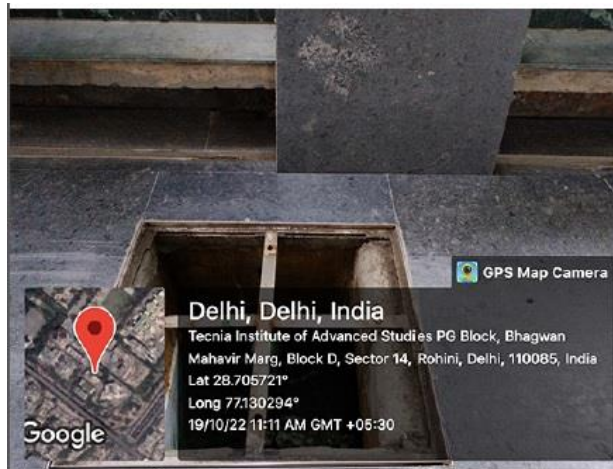
Rain water harvesting
