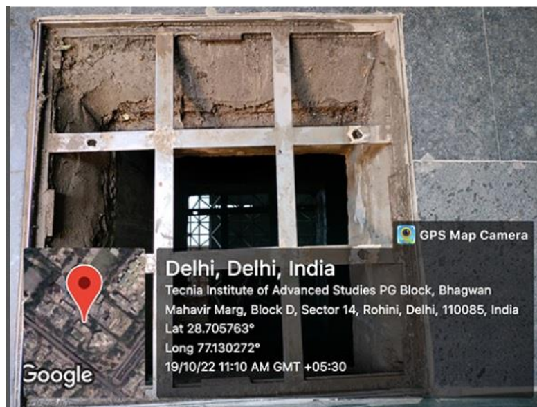
Construction of tanks and bunds
