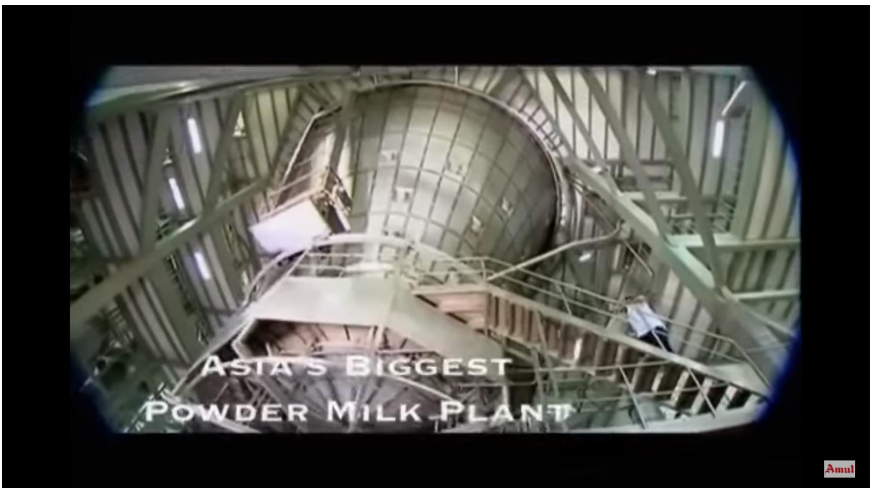
Amul Plant- Asia's Biggest Plant
